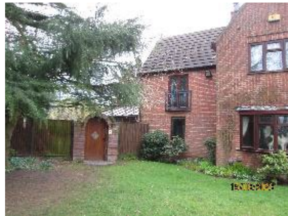
Principal elevation looking west
