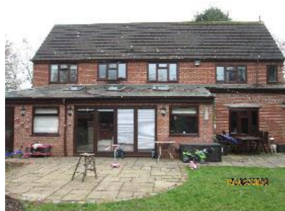
Principal elevation looking west
